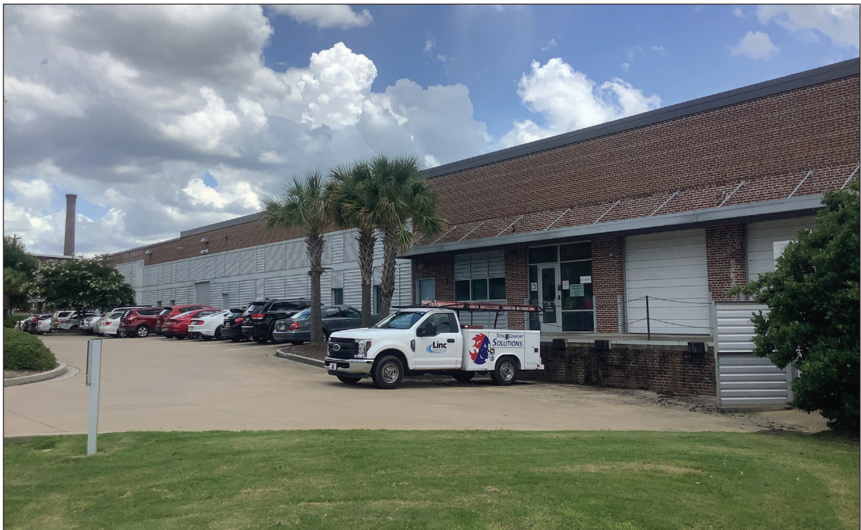
B. West End of the North Façade
