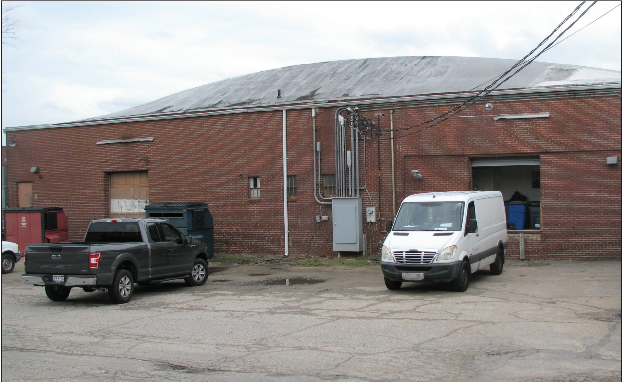
A. Warehouse, East Elevation
