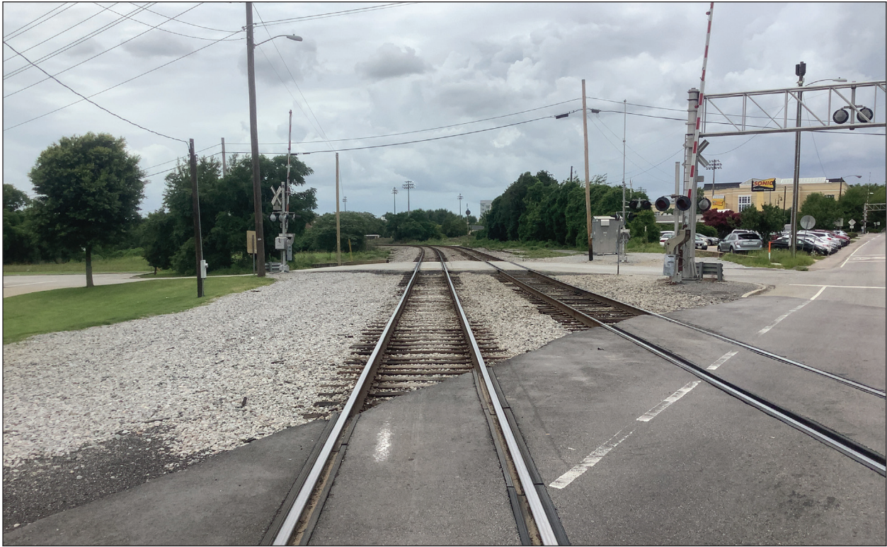
A. View Northwest
