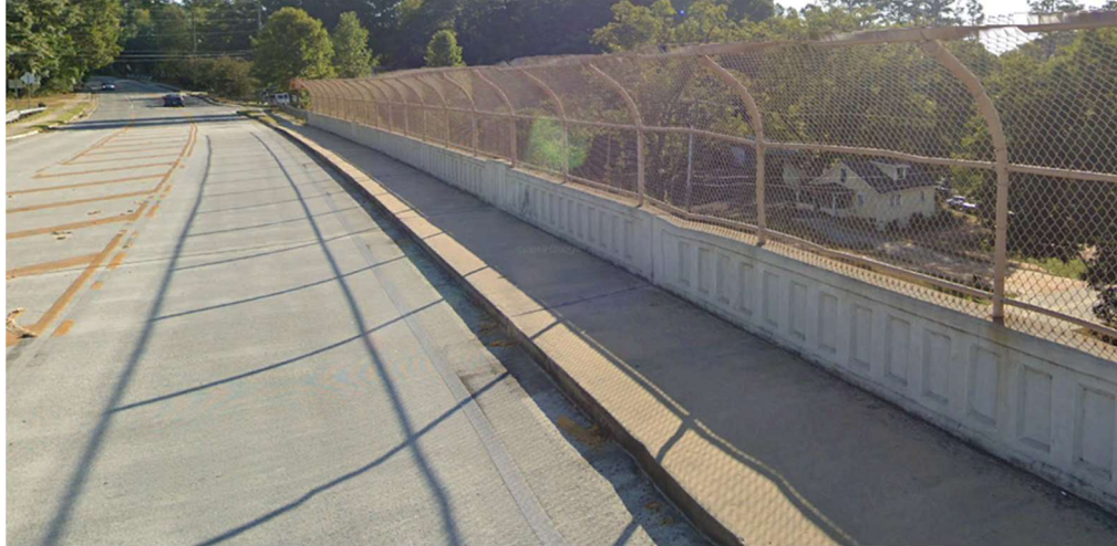
Figure 7: Sample Bridge over Railroad with Chain Link Fence and Railing with Indentions
