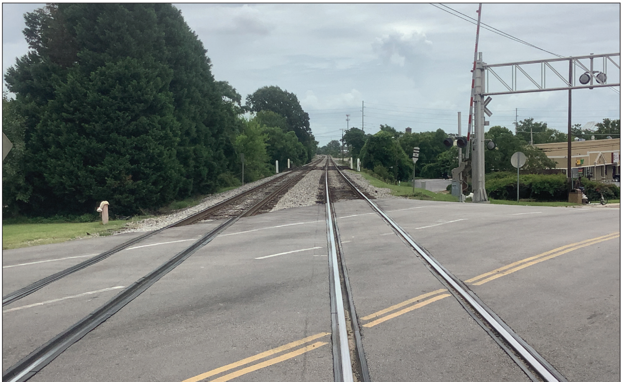
B. View Southeast
