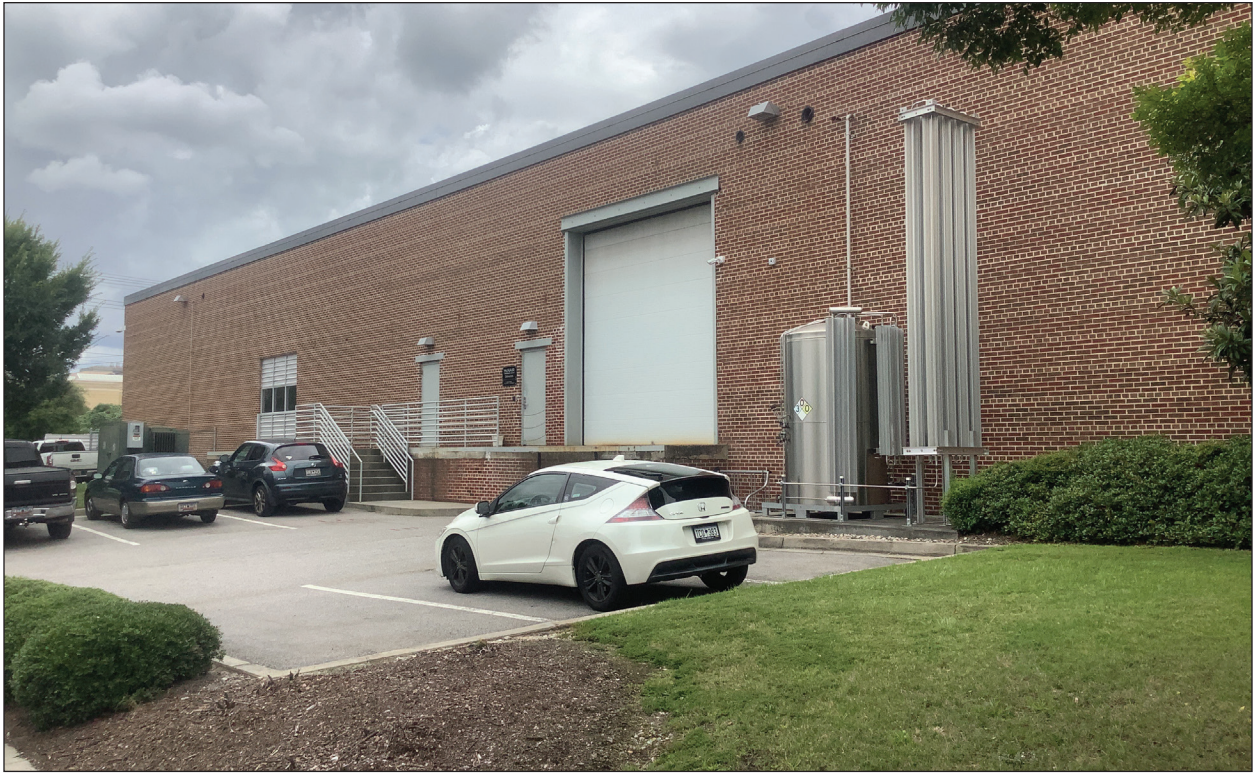
A. North End of the West Elevation
