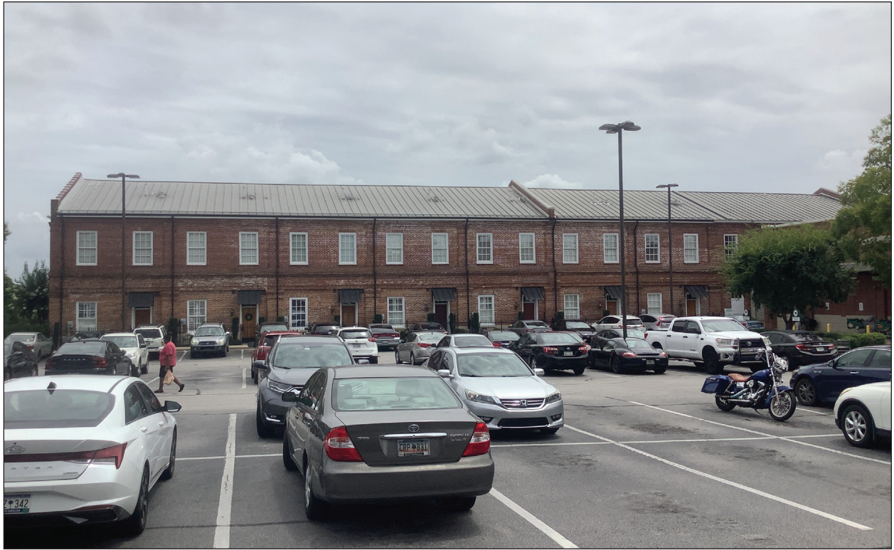
A. North Façade
