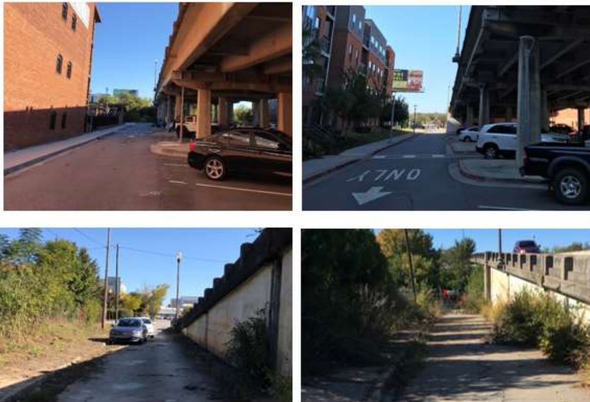
Figure 2: Clockwise from Top Left - Loop Road North of the Bridge, Loop Road South of the Bridge, NE Alley, SE Alley
