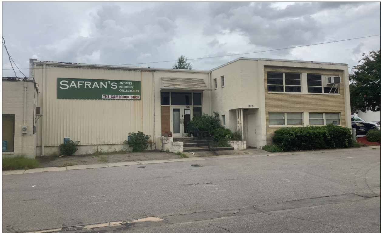
B. South Façade
