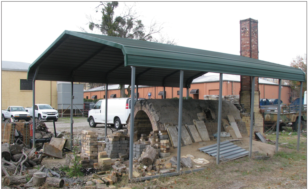
B. Kiln, View Northeast
