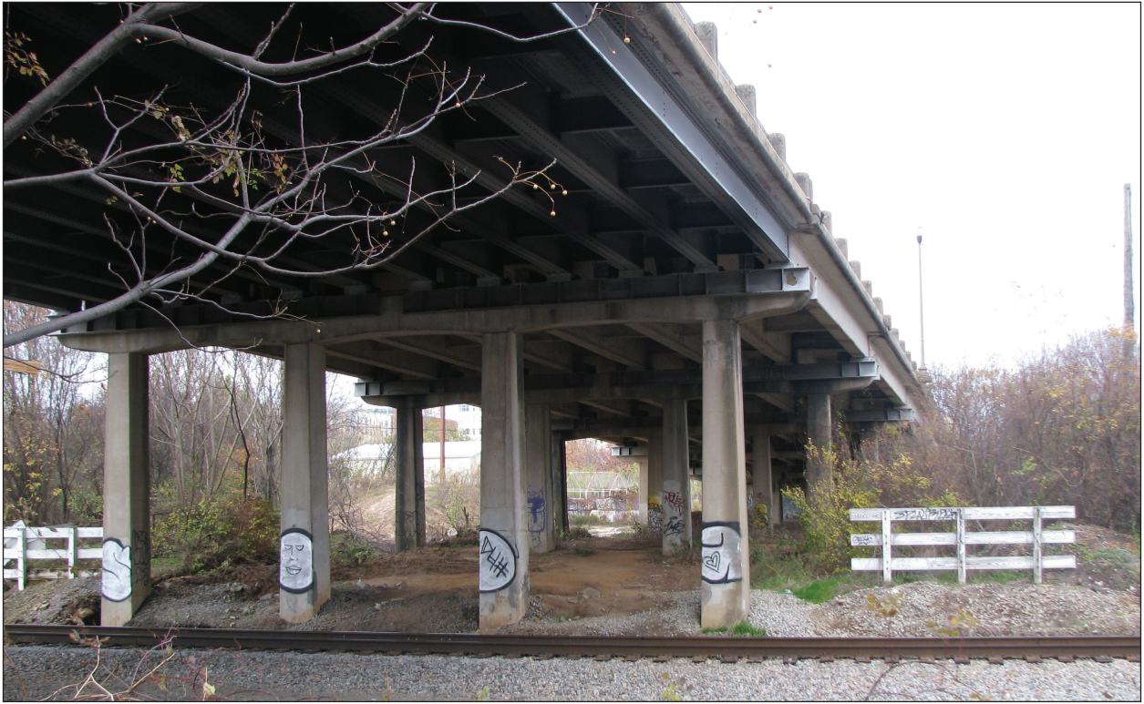
A. Bents, View Northeast
