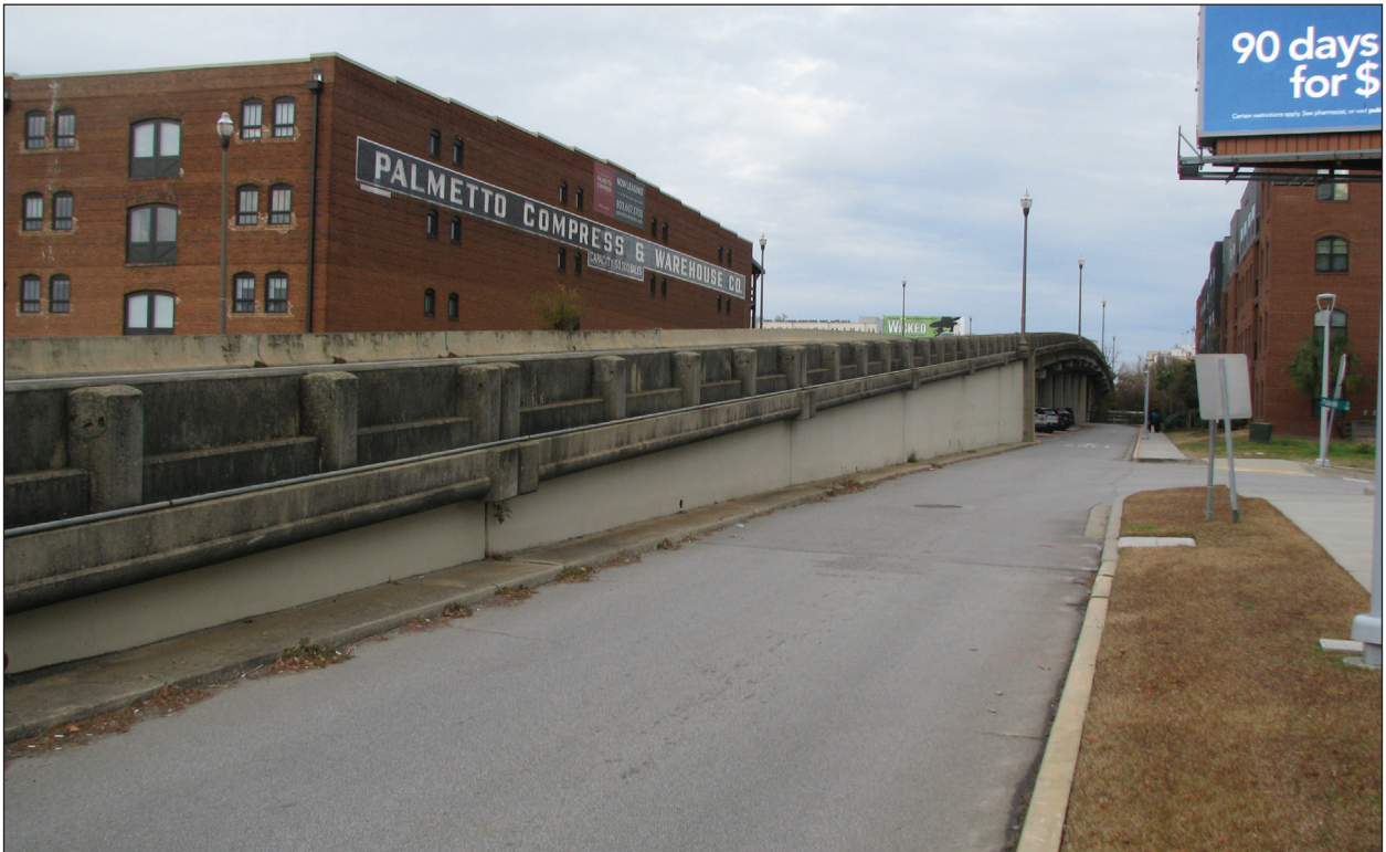
B. Railing, View Northeast
